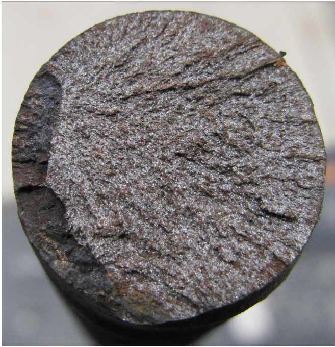
Fig. 1. A rockbolt affected by SCC. The area of initial crack growth can be seen as the dark brown section on the left hand edge of the failure surface. On this rockbolt, several cracks have initiated simultaneously and have overlapped during their growth. The remaining failure surface can be seen as speckled silver and grey, indicating brittle fracture.
