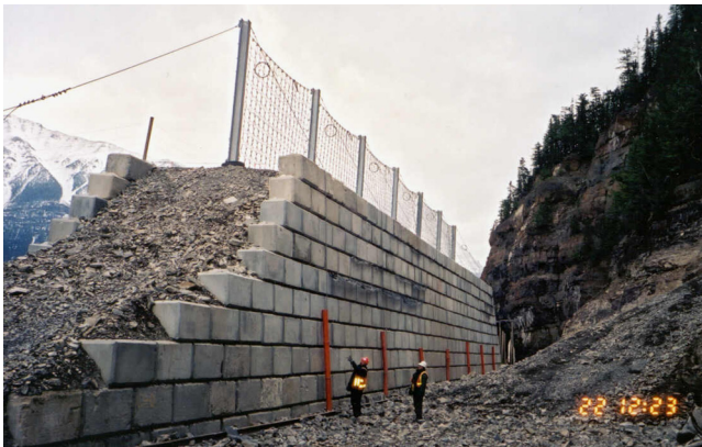
Fig. 2. Mt. Stephen – barrier constructed with concrete blocks and steel mesh fence to contain rock falls and snow avalanches.
