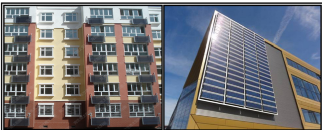
Fig. 1. Solar hot water collectors and photovoltaic panels on building facades.
