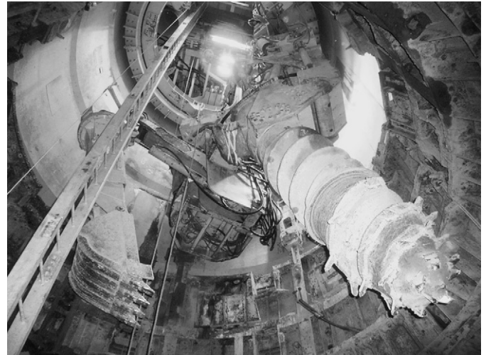
Fig. 2. Photograph of the roadheader in the Ventilation Shaft.
