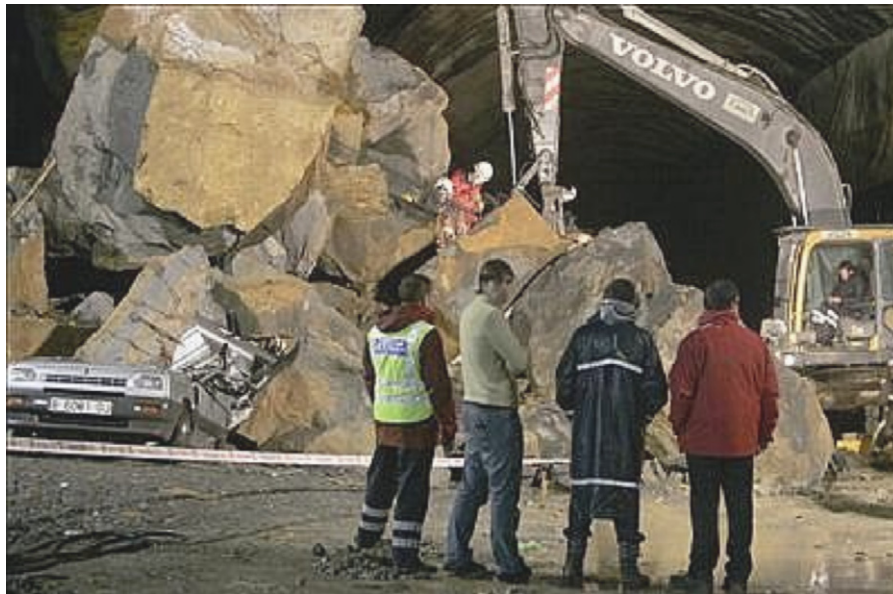
Fig. 2. Rockfall in late 2005 at a tunnel mouth in Northeast Spain resulting in one fatality [7].
