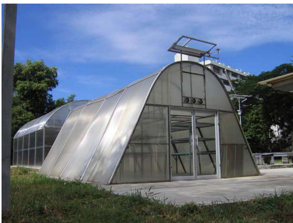
Fig. 2. The developed greenhouse solar dryer.
