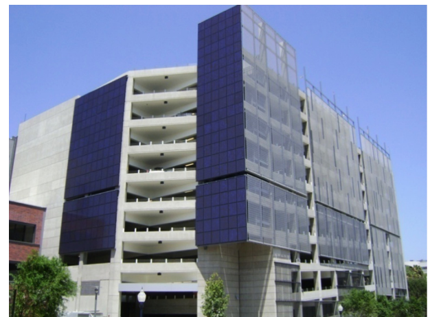
Fig. 1. Solar panels mounted vertically on the walls of a building in San Diego, USA [15].
