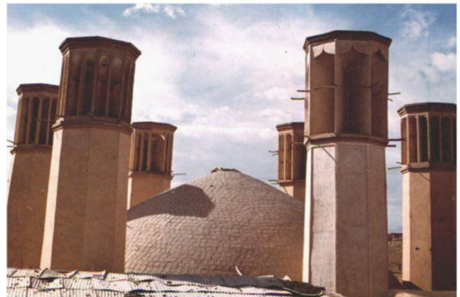
Fig. 1. A city cistern in Yazd with six wind towers.
