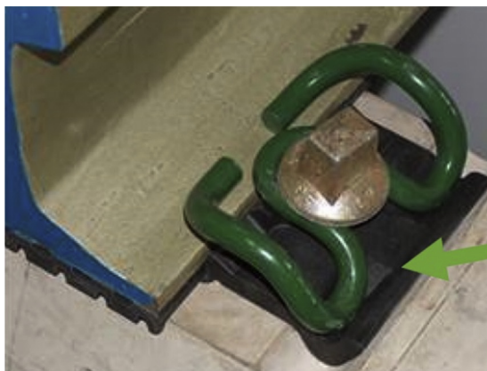
Fig. 1. Railway fastening system [24].
