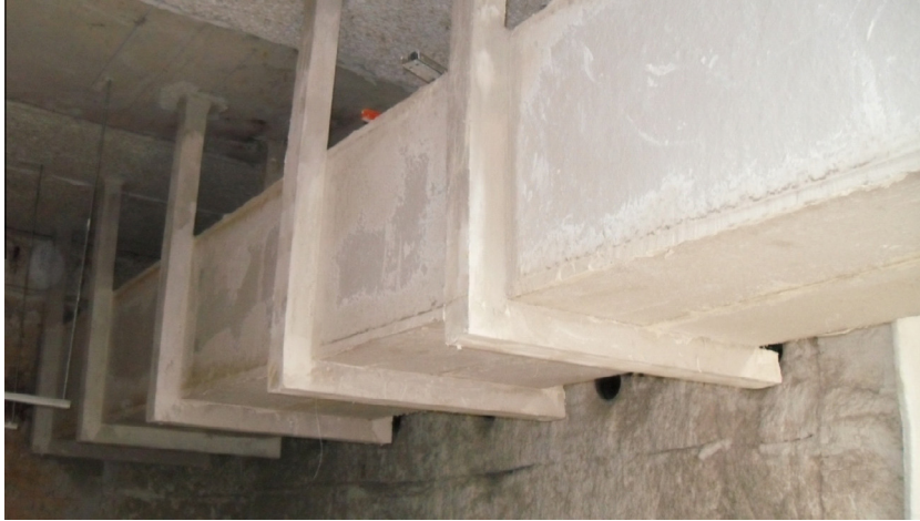
Fig. 1. Assembly of a horizontal smoke extraction conduit.
