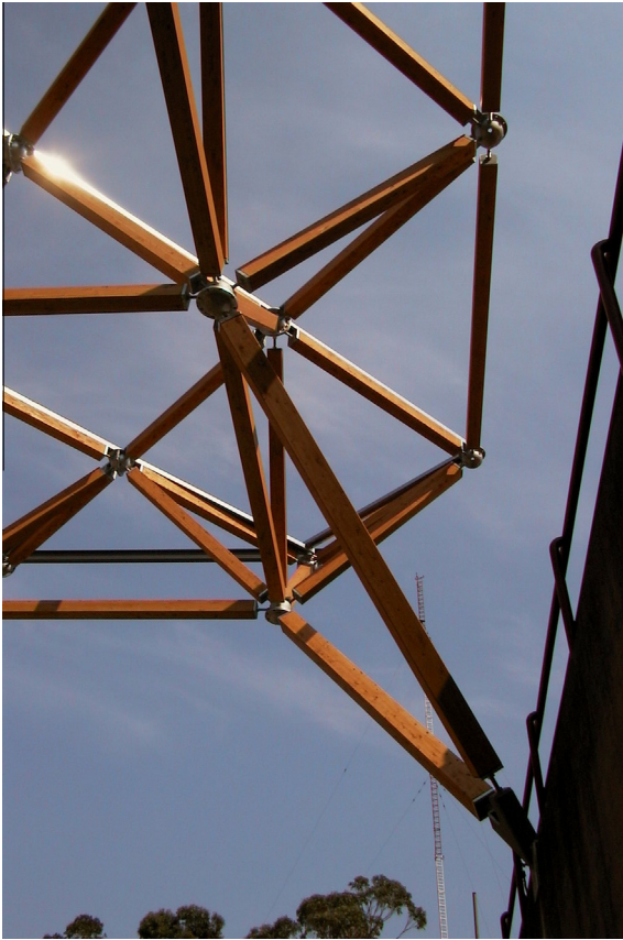
Fig. 1. Spatial mesh of hollow bars made with glued laminated timber and joints made of threaded bars glued with epoxy resin.
