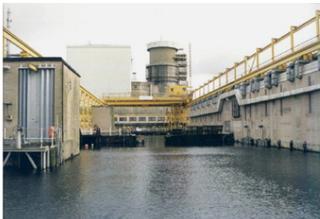
Fig. 1. First Generation Magnox Storage Pond (Hastings et al., 2007).
