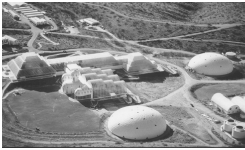
Fig. 1. Aerial photograph of the Biosphere 2 facility, showing rainforest, savannah/ocean/marsh to desert (top section of glass space frame), human habitat and agriculture (barrel vaulted structure middle right), two variable volume “lungs” (white domes) and external energy center (bottom right). The research and development complex is at the top of the photo (photo by Gill C. Kenny).
