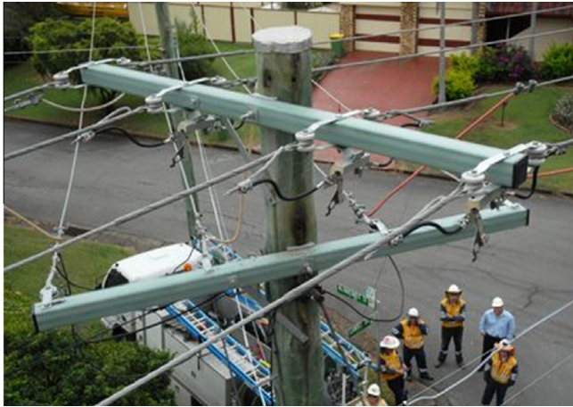
Fig. 1. Pultruded FRP tube as power pole cross-arms [13].
