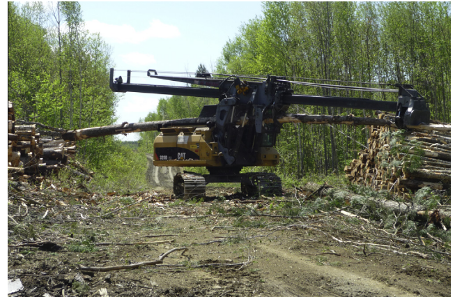
Fig. 1. A stroke delimeter generally processes one tree at a time by cutting off branches and the top above a specific merchantable diameter.
