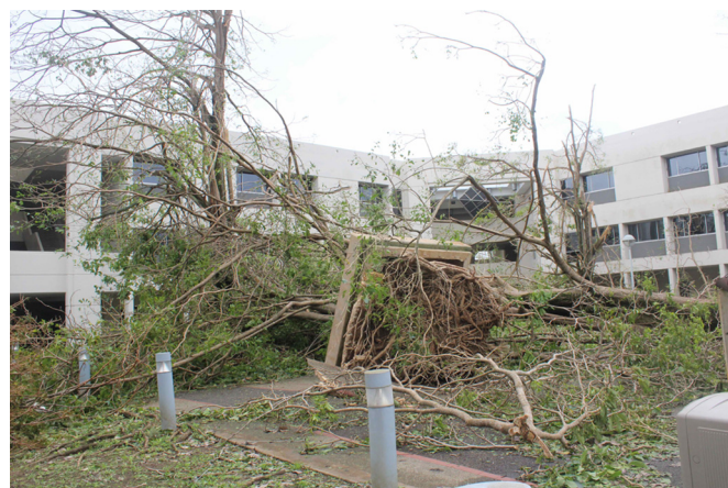
Fig. 1. Inner patio of the Natural Sciences Building at UPR, Rio Piédras following Hurricane Maria. Credit: José García-Arrarás
