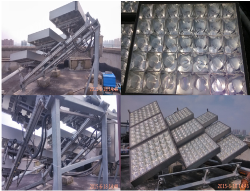
Fig. 2. The physical configuration of the CPV system.
