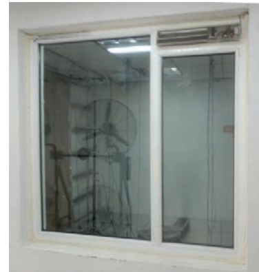
Fig 2. The new ventilated window
