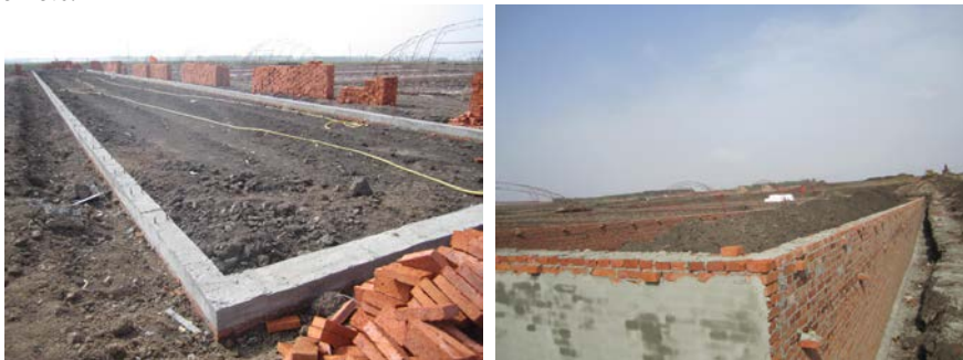
Figure 1 brick structured greenhouses in construction
