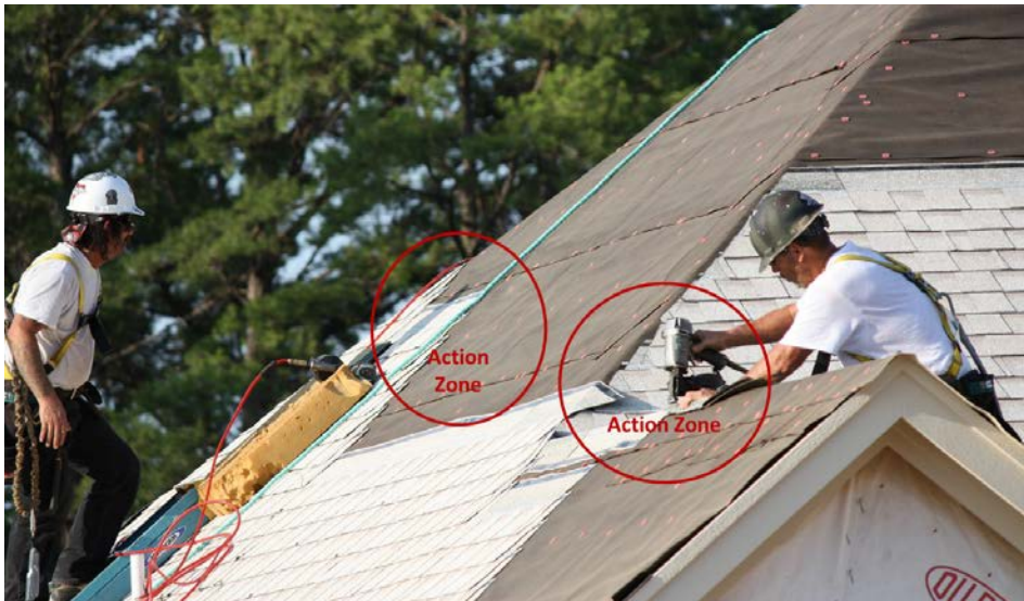
Figure 1. Each nailer is working in their own Action Zone.
