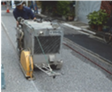
a) Asphalt surface cutting site
