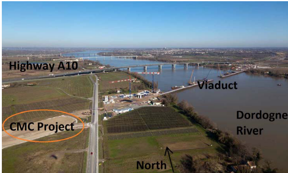
Figure 1: Aerial picture of the site, from COSEA
