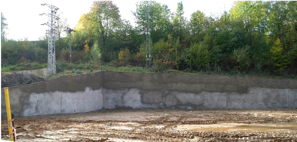
Fig. 1 View of the wall excavation.
