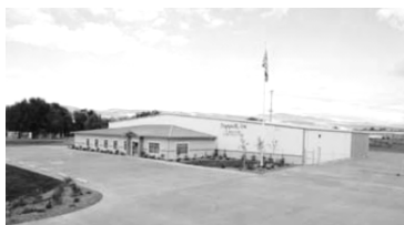
a. Concrete floor, driveway and warehouse built by Macro polymeric Synthetic FRC [13]
