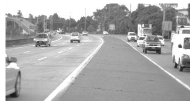
c. Concrete pavement grade replaced by FRC at Hex ham, Australia [14]
