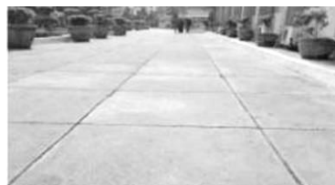
b. Pavement with Steel FRC [1]
