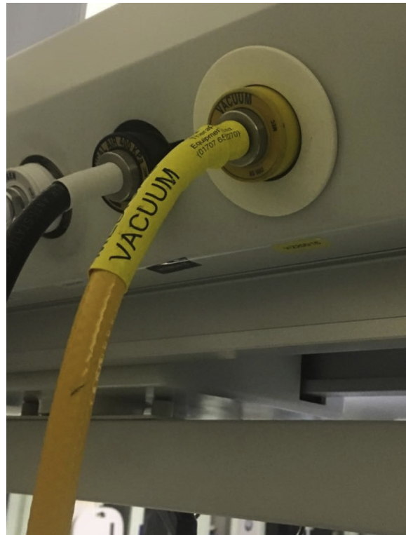
Figure 1 Suction vacuum wall inlet.
