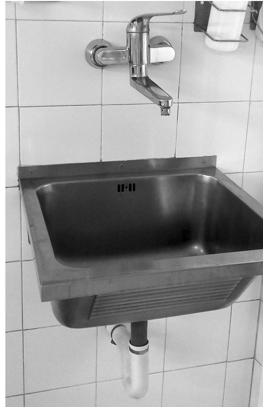
Figure 1. A sink before the intervention.
