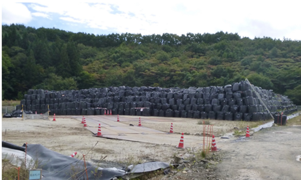
Fig. 1. Photograph of a typical waste storage study site within Kawamata (Date District), Fukushima Prefecture, prior to final waterproofing of the structure.
