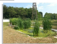
Aerated Free water surface (FWS)
