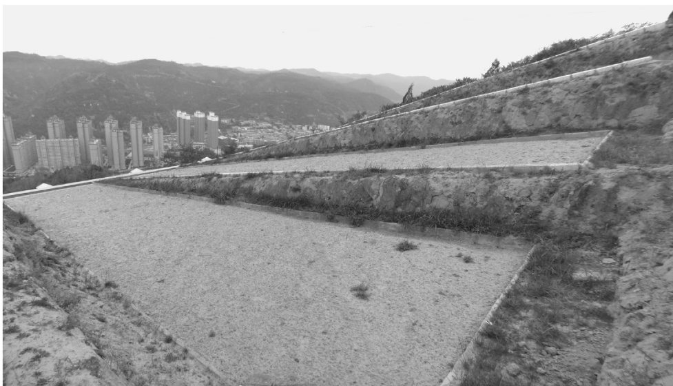
Fig. 1. Recently established 20 m long plots with different slope gradients on a landscaped hillslope area at the Ansai Research Station installed to re-establish the situations used in the 1985–1992 experiments.
