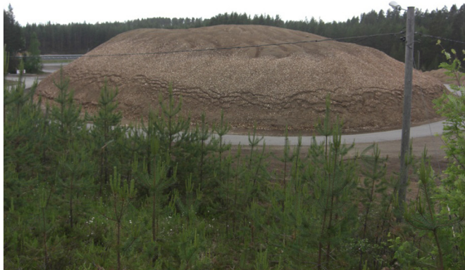
Fig. 1. Snow storage (about 25,000 m 3 ) insulated with sawdust, Vuokatti, Finland, 2013.
