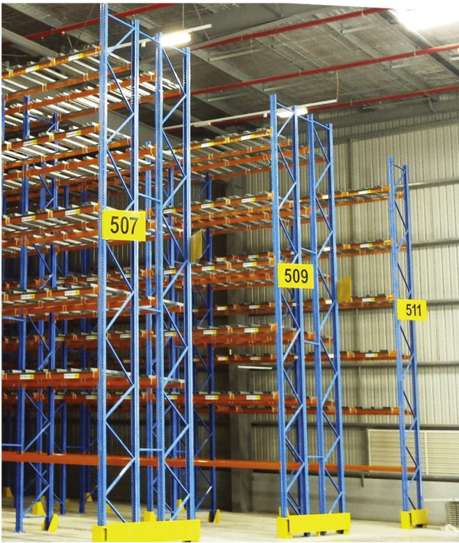
Fig. 1. Typical upright frames.
