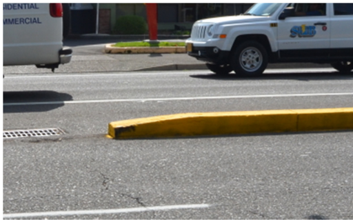
Fig. 2. Concrete median/curb struck by the 2009 International ambulance. The initial height is 10 cm and the full height is 19 cm.
