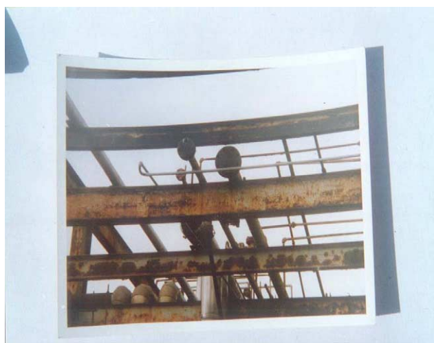
Fig. 2. Jumper line was connected to PVH line (left) and RVVH line (right, larger diameter).
