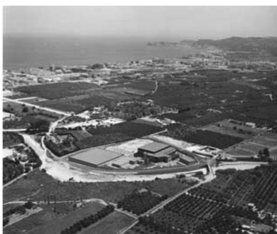
Fig. 2. Aerial view of the desalination plant.
