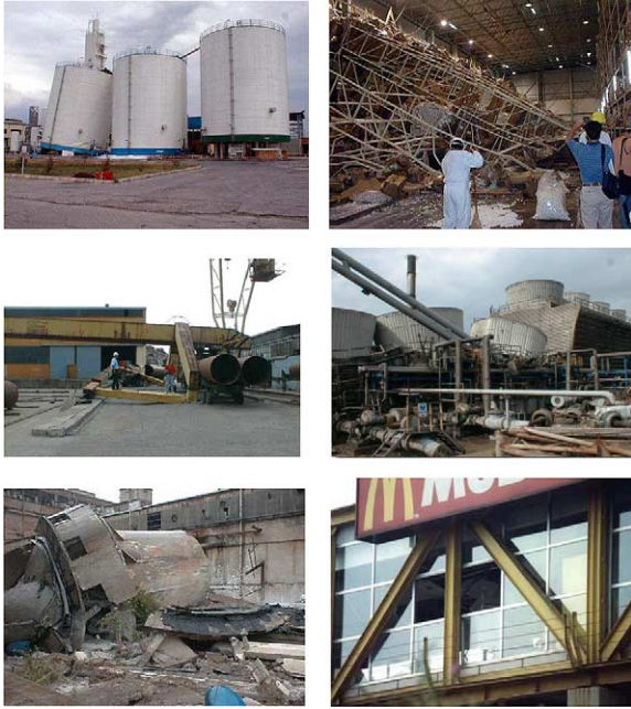
Fig. 1. Samples of the fractured steel construction in 17 Agust and 12 November 1999 İzmit.
