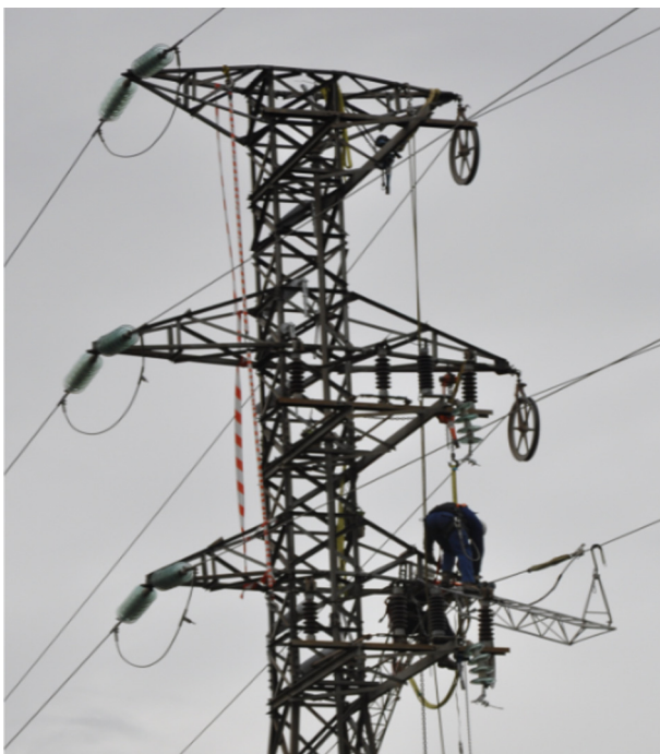
Fig. 1. Stringing the gap-type conductor.
